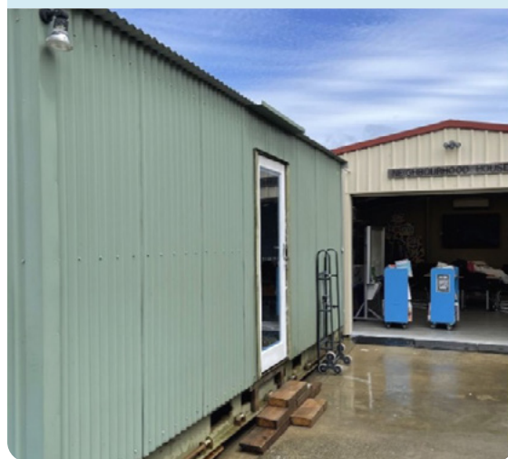
Shipping container in place
